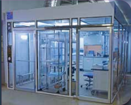
Los Angeles Clean Room
